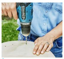
**Step 11** Remove the ears and drill two pilot holes per ear within the marks you have made on each stool. Position ears so that legs do not obstruct the pilot holes.
