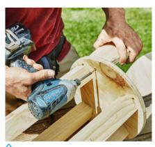
Step 12: Placing the stool on its side, apply some glue to the ear and use the 45mm screws to fasten the ears into place. Repeat for other ear.
