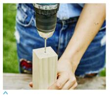
**Step 6:** Mark in pencil where legs are to be positioned on seat. Using a 1/4 drill bit, drill pilot holes in the centre of each leg.
